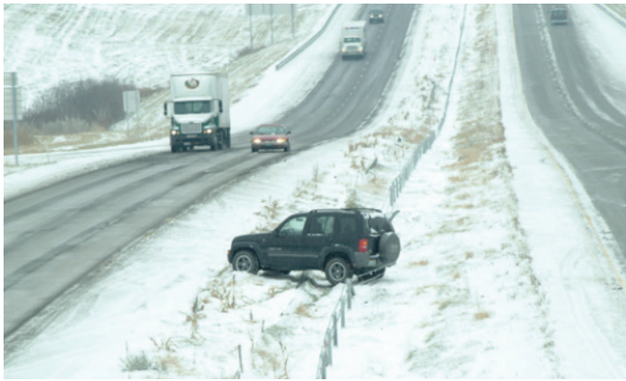
Figure 8. Ms. Bernskoetter's Vehicle Snagged by a Cable Median Barrier on I-70 in Missouri
